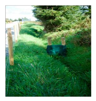
Figure 3-5: Silt trap across grassed swale
