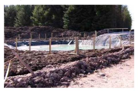
Figure 3-9: Lined Settlement Lagoon for Concrete Washout Facility
